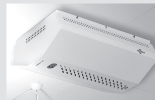
The finished ceiling-mounted installation.
