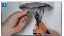
Slide the metal coil on the hose slightly upwards and cut the hose as shown.
